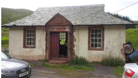
Meter House before and after renovation
